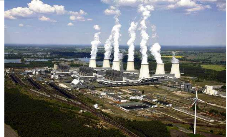
Germany's Jämschwalde power plant, one of six sites to receive EU funding for CCS projects
